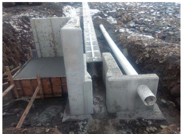
This is a construction photo of the entrance of the steep pass fishway. The attraction water/downstream bypass pipe is to the right and the slab to the left is where the eel pass will be installed.
