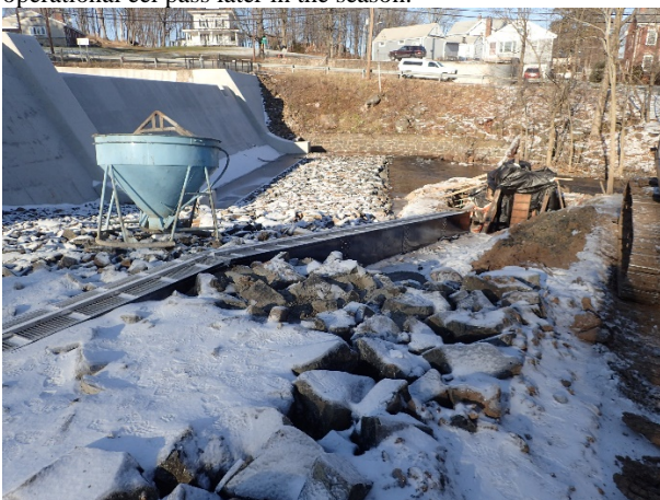
This is a construction photo of the steep pass fishway. There is a grating locked down on the top of the fishway for safety and the sides were being backfilled with rip rap when this photo was taken. The dam's spillway can be seen to the left. The attraction water pipe is buried alongside the steep pass.
